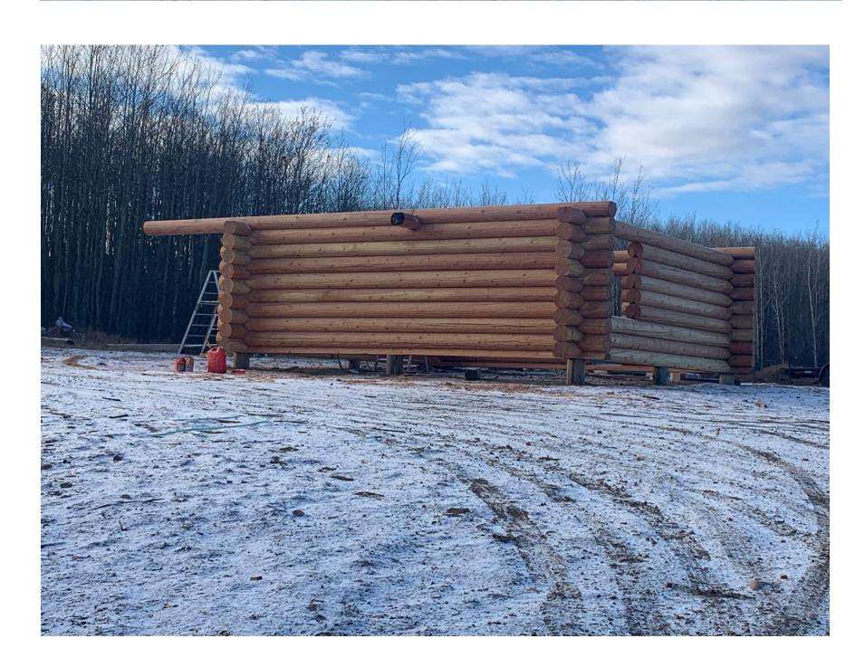
Embark on an enchanting journey with our meticulously crafted 24x24 log cabin, fashioned from premium dry Douglas fir logs. Immerse yourself in the captivating allure of 12-inch diameter scribe fit logs, showcasing intricately hand-cut saddle notch corners. This exceptional structure is prepared for immediate delivery or can be securely stored until your preferred spring arrival.
